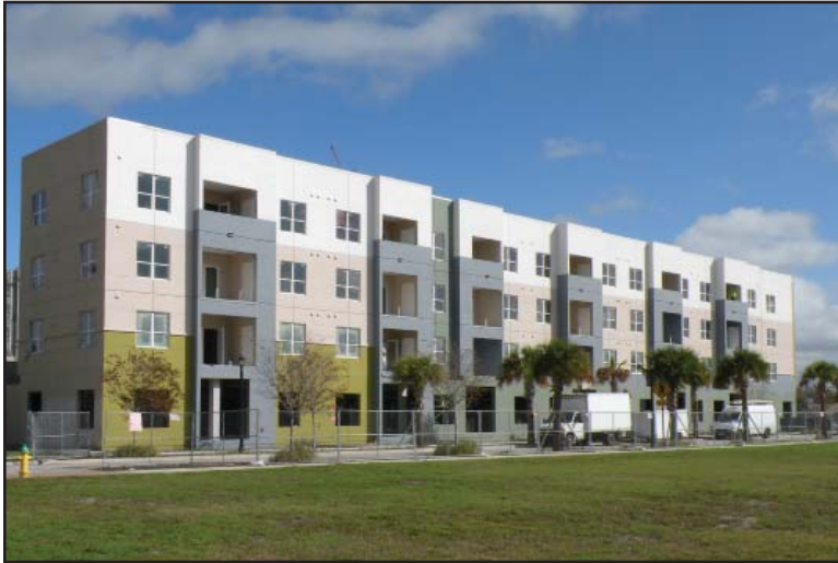
Progress on the Trio building
