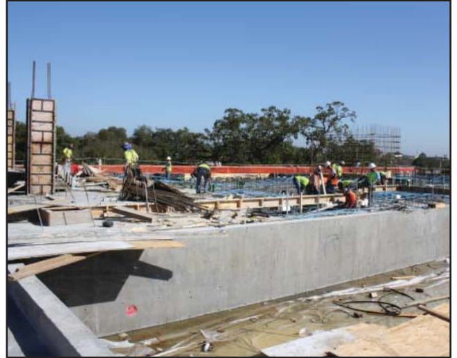
Construction on the Reed's 4th floor pool deck
