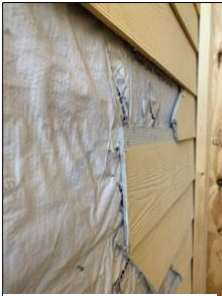
Cement board siding fastened to building paper leaving no gap for drainage.
